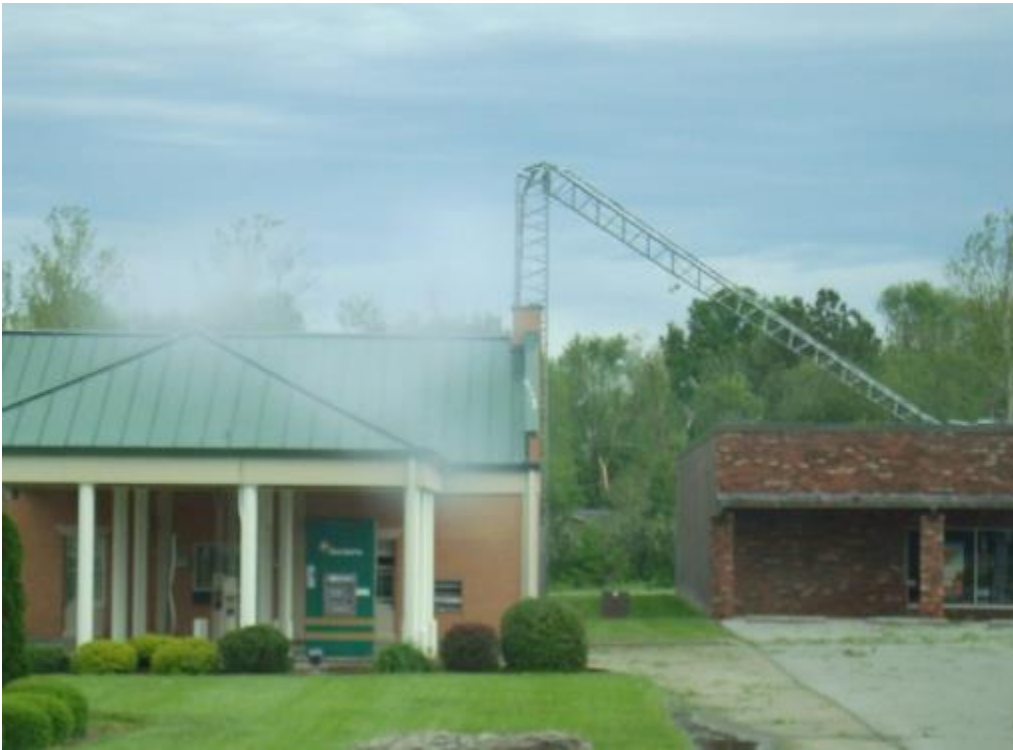
Signs were blown out...
